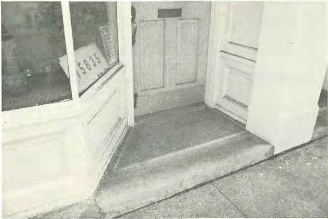
Sheltered entry doors and paneled bulkheads - nice features from the commercial past.
