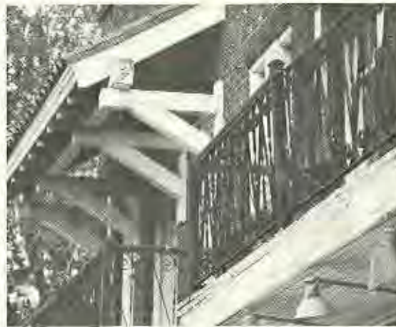
A variety of balconies are to be found on Lakewood's structures.
