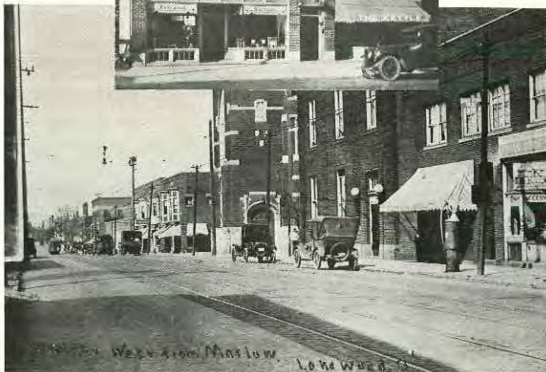
Photos taken of Lakewood in the early 20's and 30's reveal many architectural details that still remain today.
