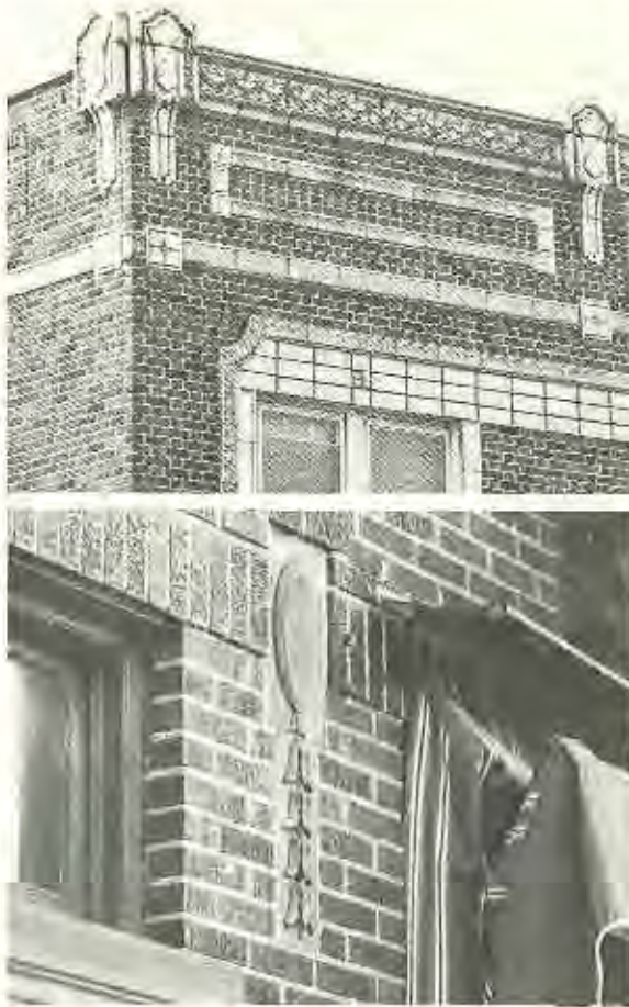
Terra cotta (above) and brick trim work is a characteristic of many of Lakewood's commercial buildings.
