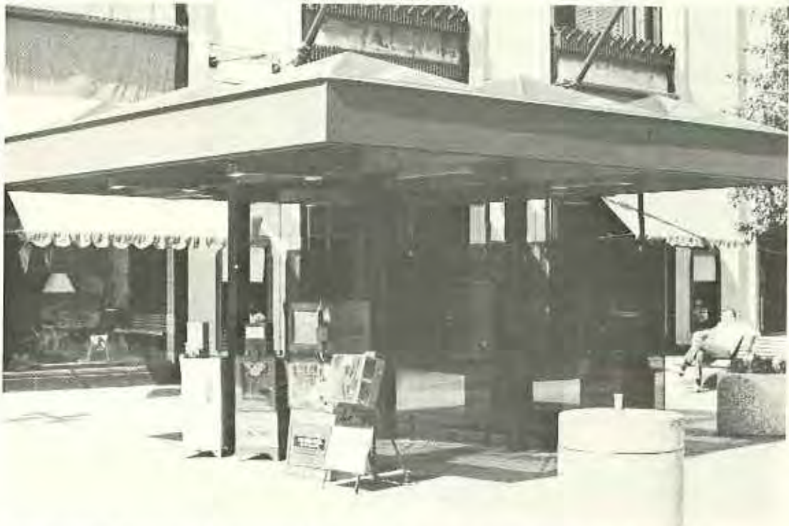
Any right-of-way work should be understated so as to coordinate itself with the storefront renovation work.
