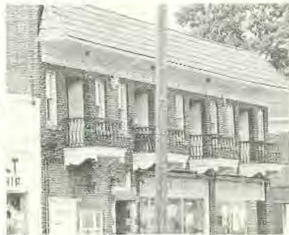
Balconies can form a pleasant repetitive pattern.
