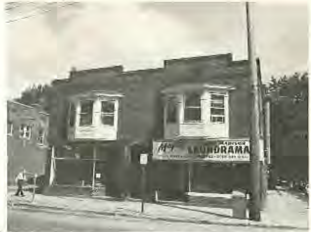
Bay windows and active parapet walls are common Lakewood commercial area features. They need preservation - and sometimes restoration.
