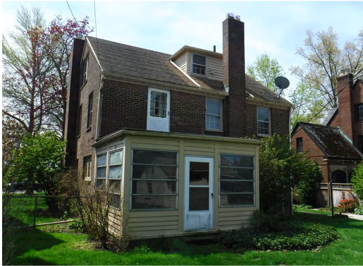
EXISTING PHOTO VIEWING SOUTHWEST
