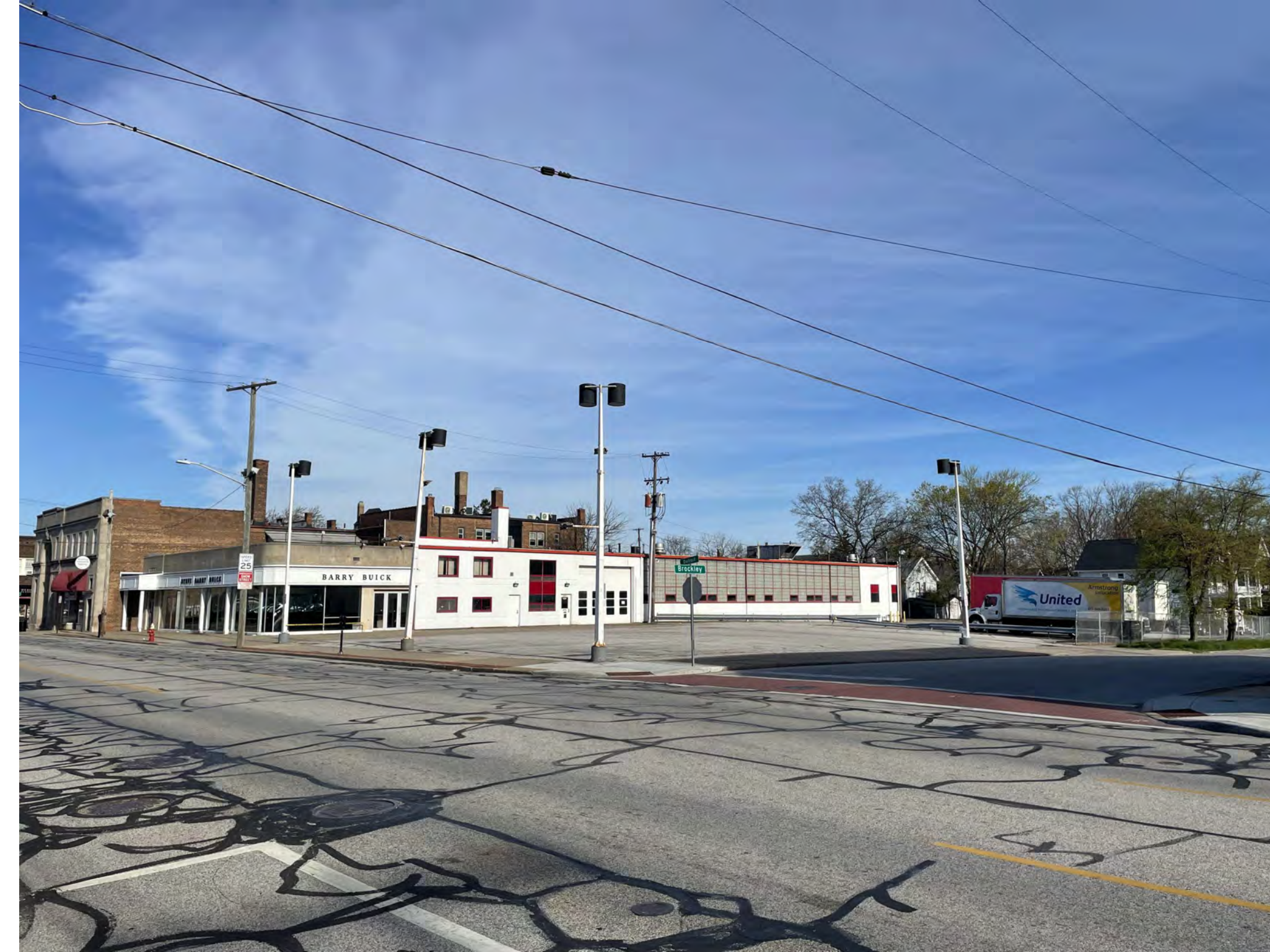
2. Brockley Avenue & Detroit Avenue Intersection
