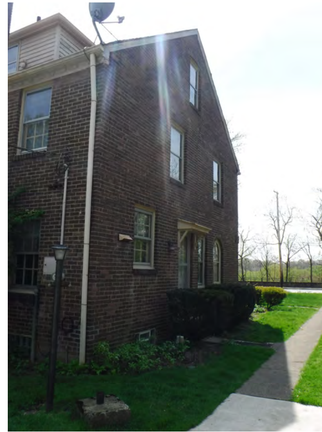
EXISTING PHOTO VIEWING SOUTHEAST
