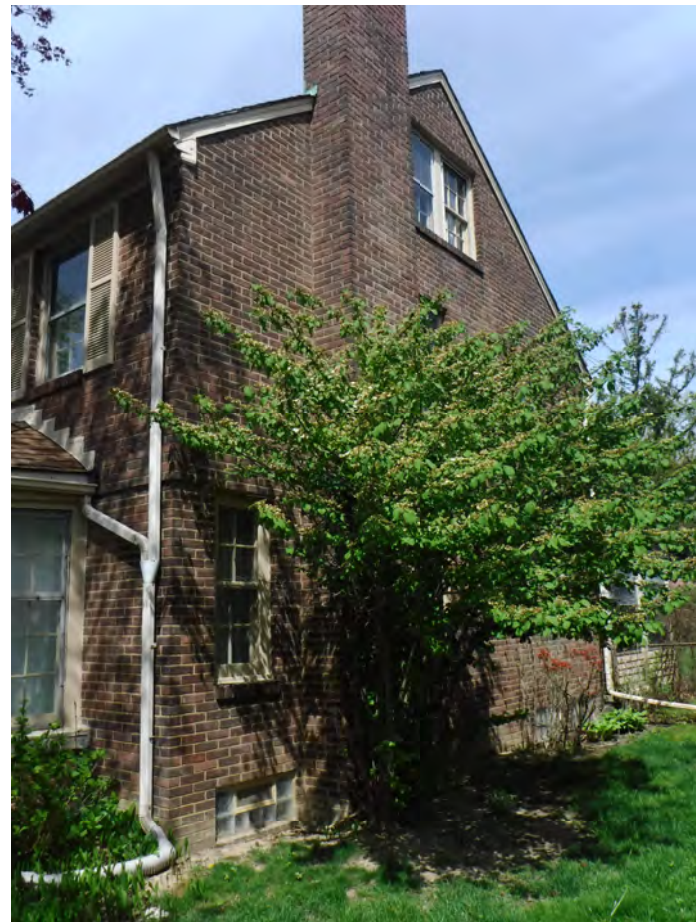
EXISTING PHOTO VIEWING NORTHWEST
