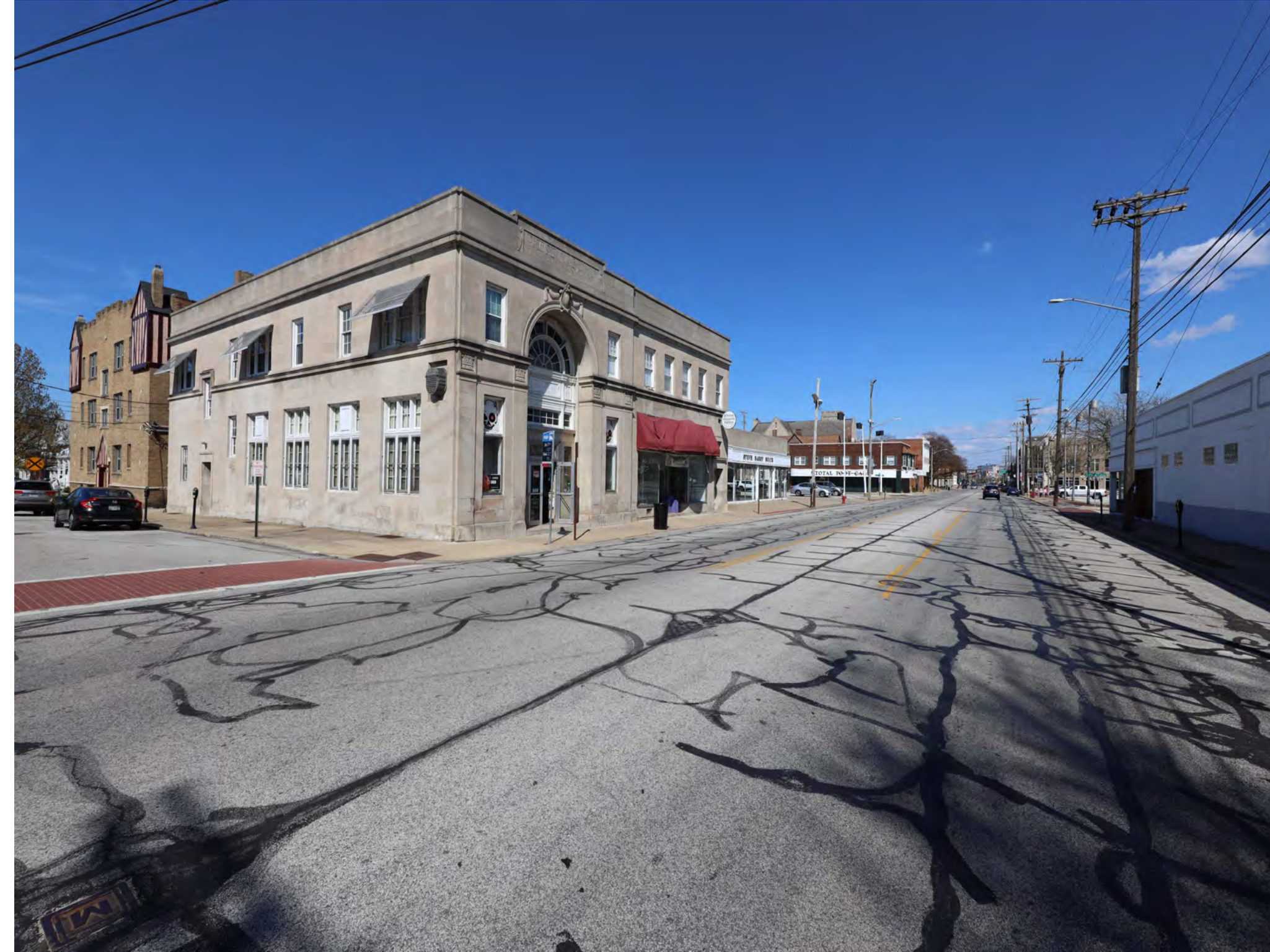
6. Cranford Avenue & Detroit Avenue Intersection Looking East on Detroit Avenue
