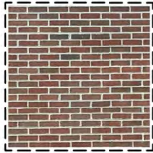
EXISTING BRICK FACADE
