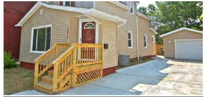
Plover Avenue rehab: exterior siding, new front steps, interior renovations, driveway, and garage.
