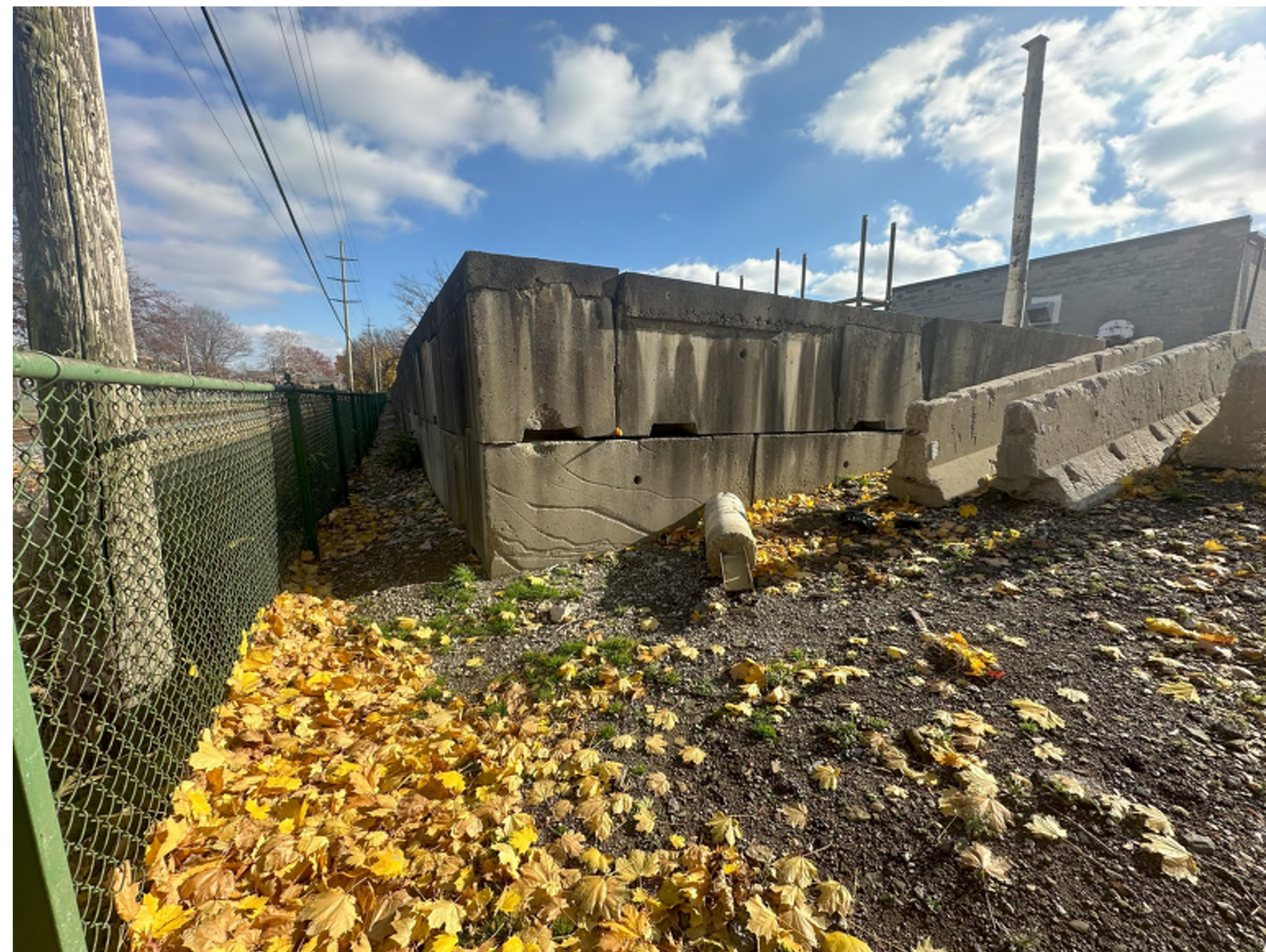
JERSEY BLOCK WALL - NORTHWEST CORNER
