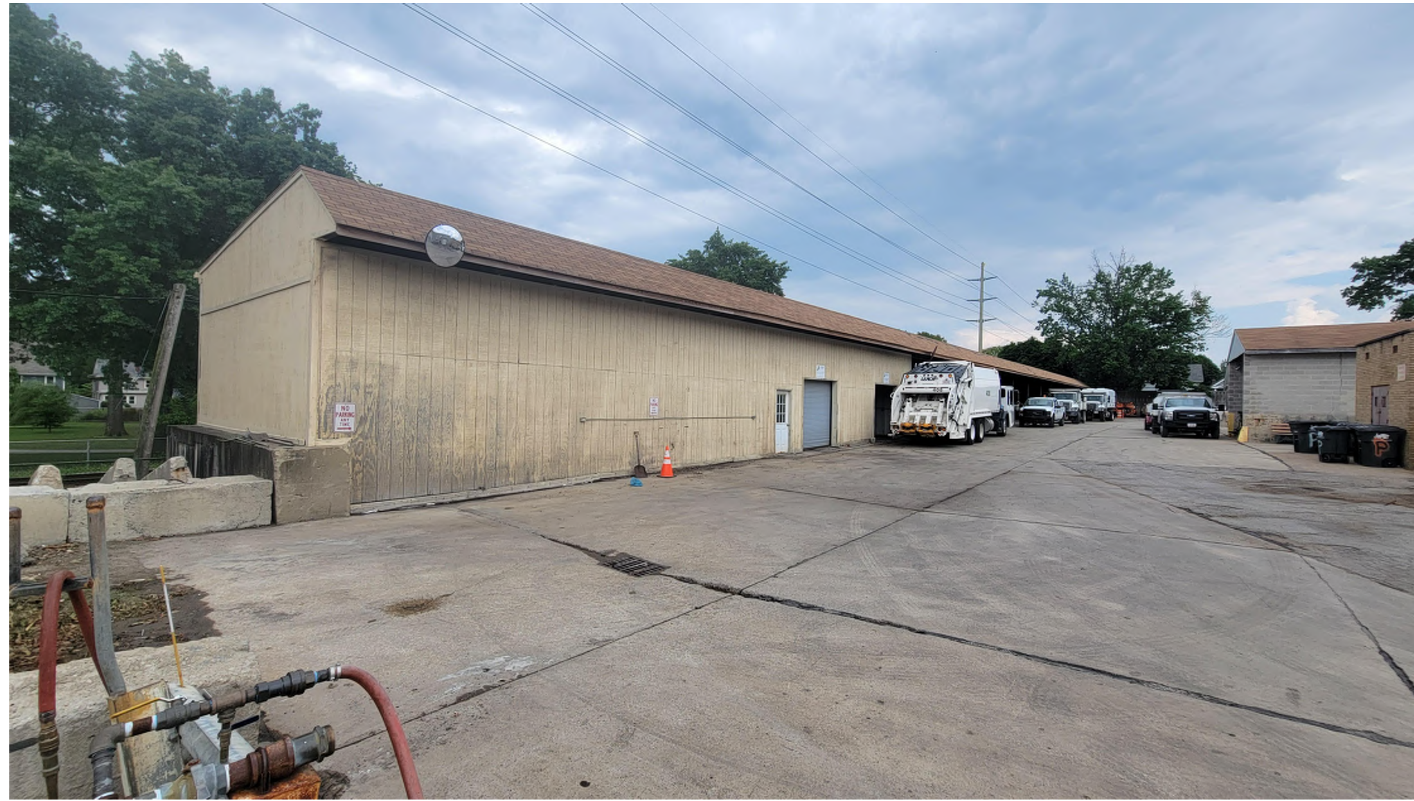
FORMER STORAGE BUILDING
