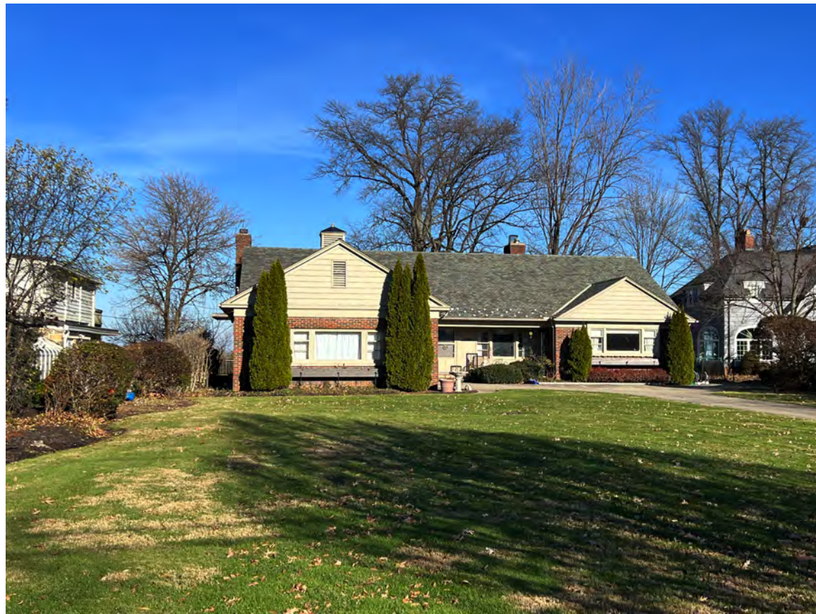
Neighbor to the East, showing the existing structure on the left
