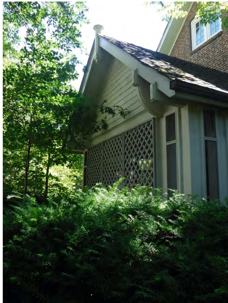
EXISTING PHOTO VIEWING SOUTHWEST
