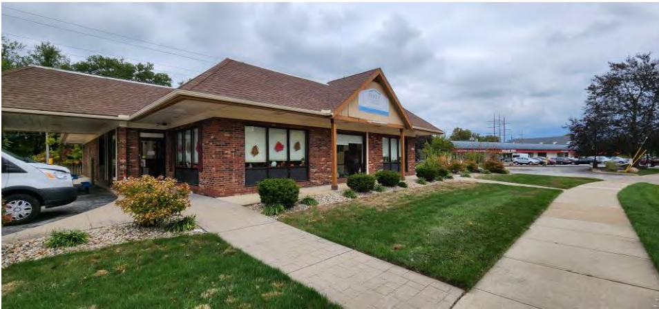
EXISTING BUILDING FROM SOUTHWEST
