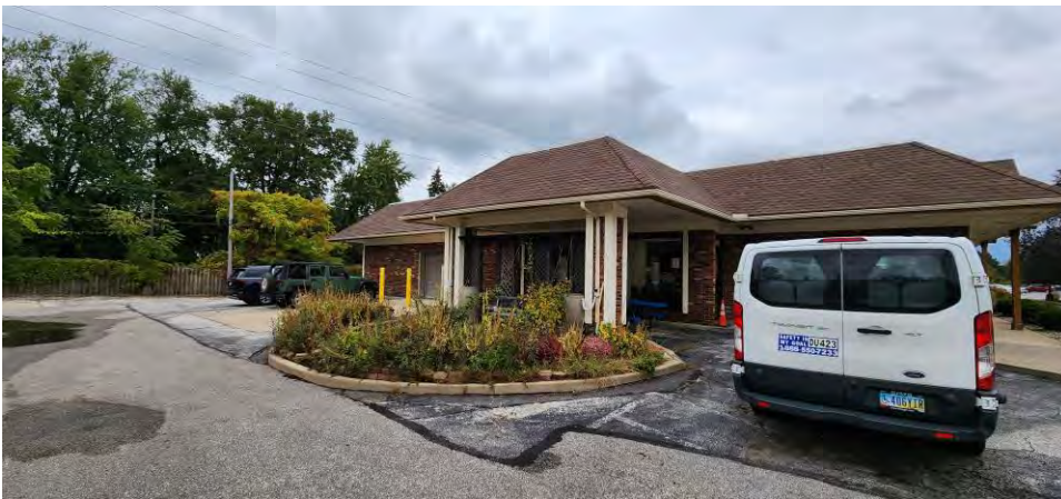
WEST SIDE WITH EXISTING CANOPY
