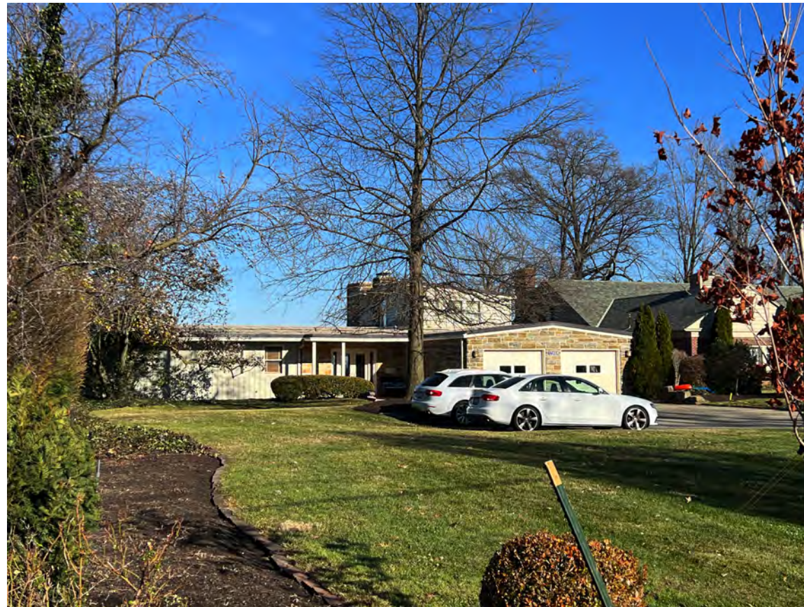
Existing structure to be demolished
