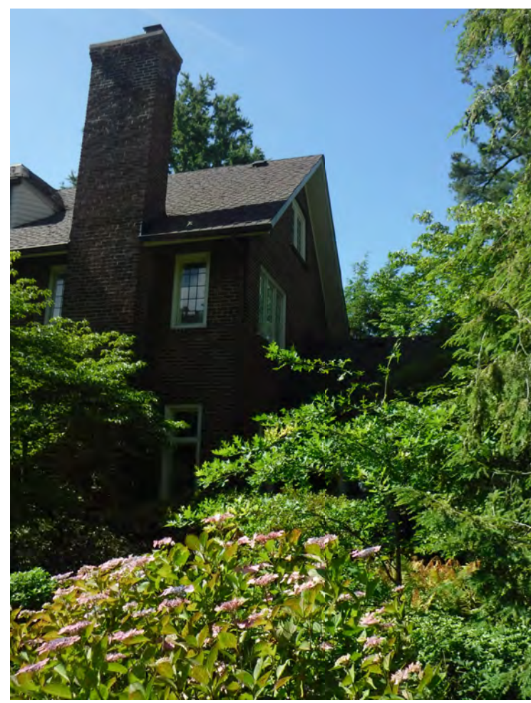
EXISTING PHOTO VIEWING NORTHWEST
