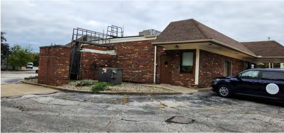
REAR OF EXISING BUILDING (EXIST LADDER TO BE REMOVED)
