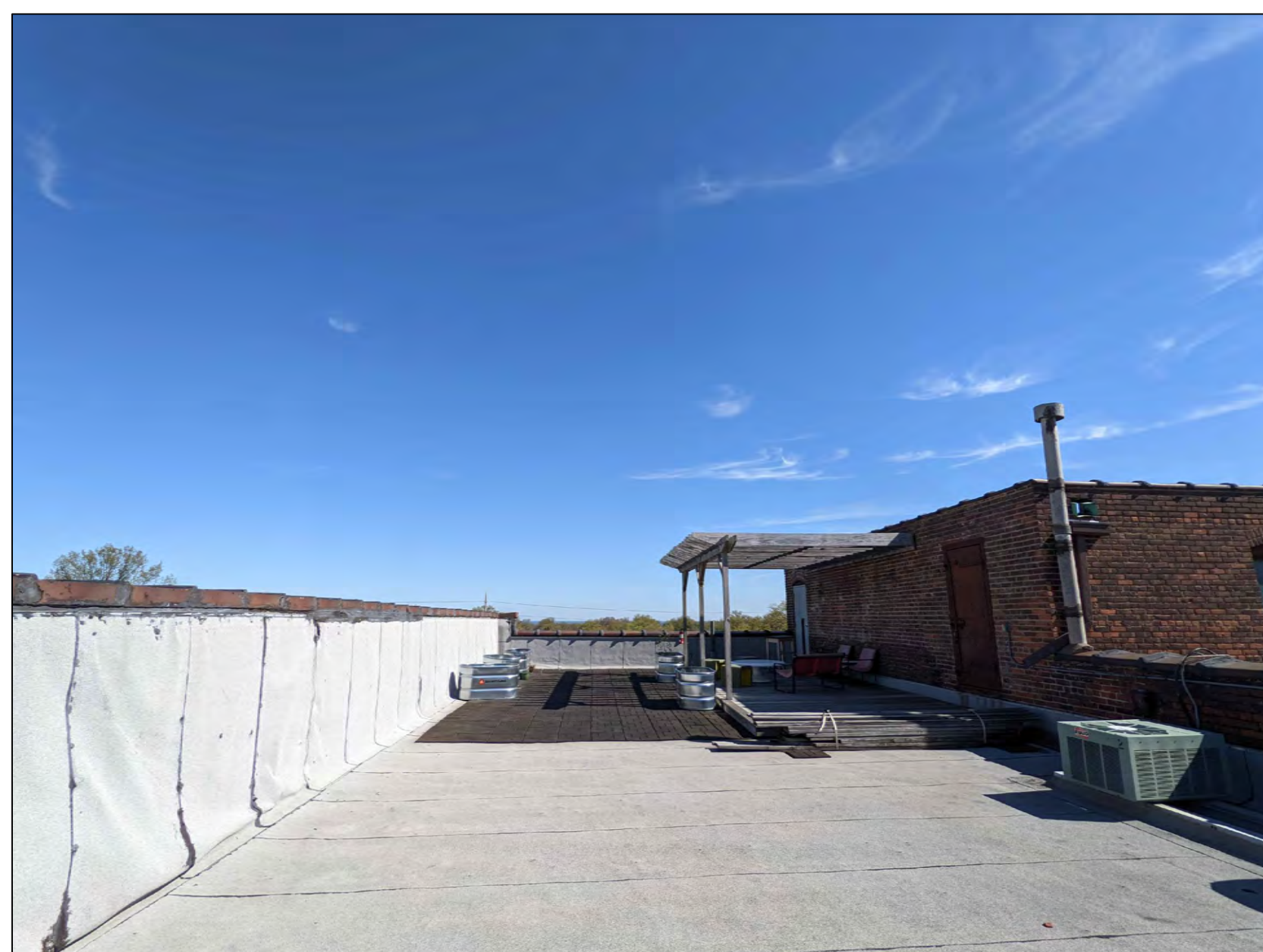
Existing Accessible Roof
