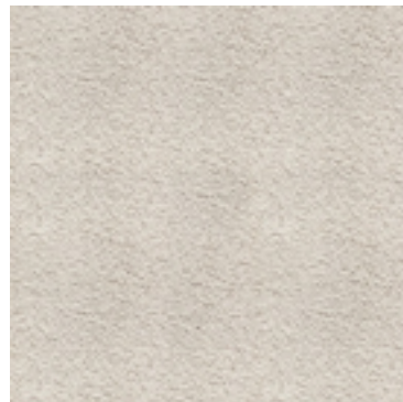
Existing EIFS Cladding
