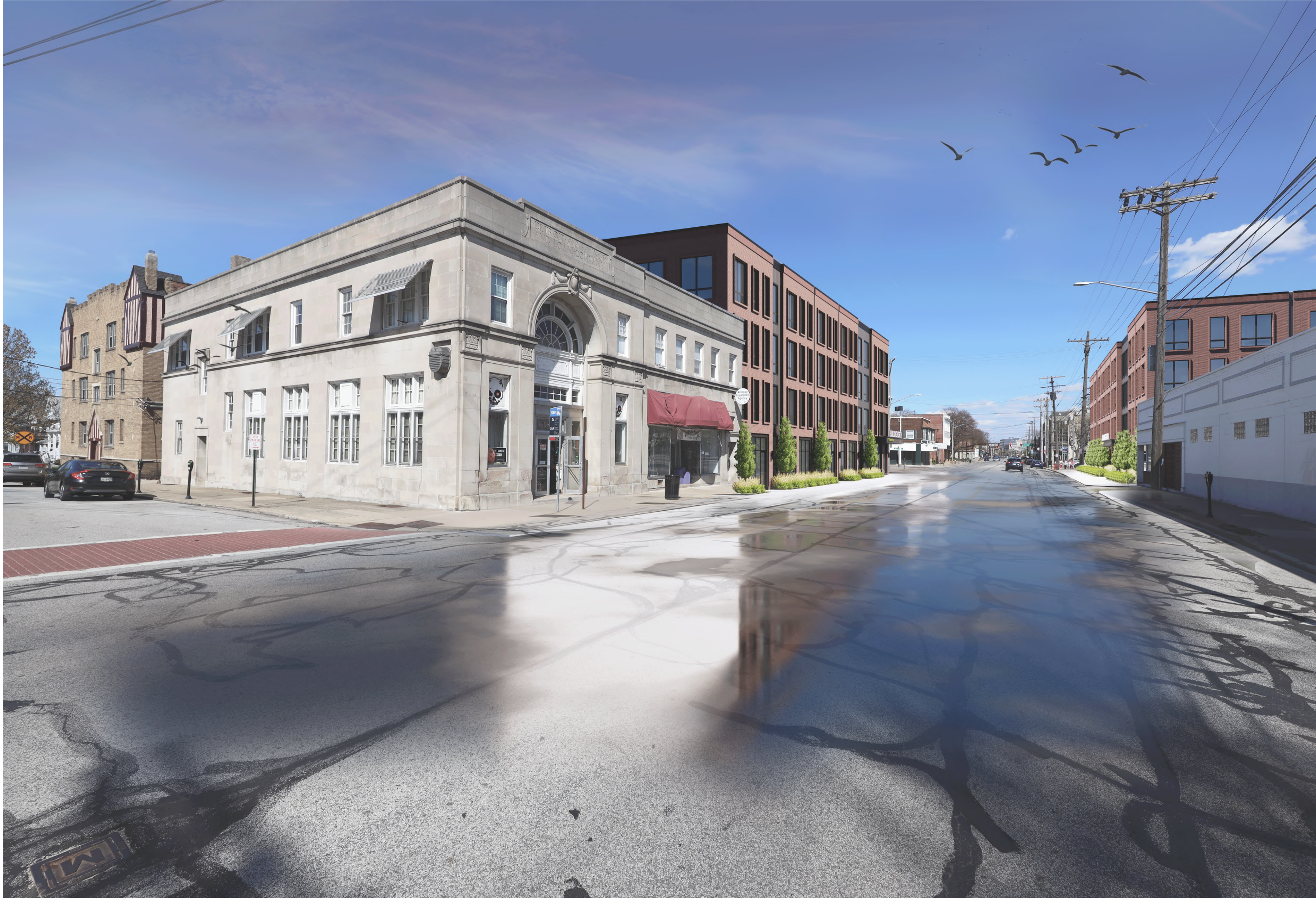
1. BUILDING NORTH & SOUTH - CORNER OF DETROIT AVENUE & CRANFORD AVENUE
