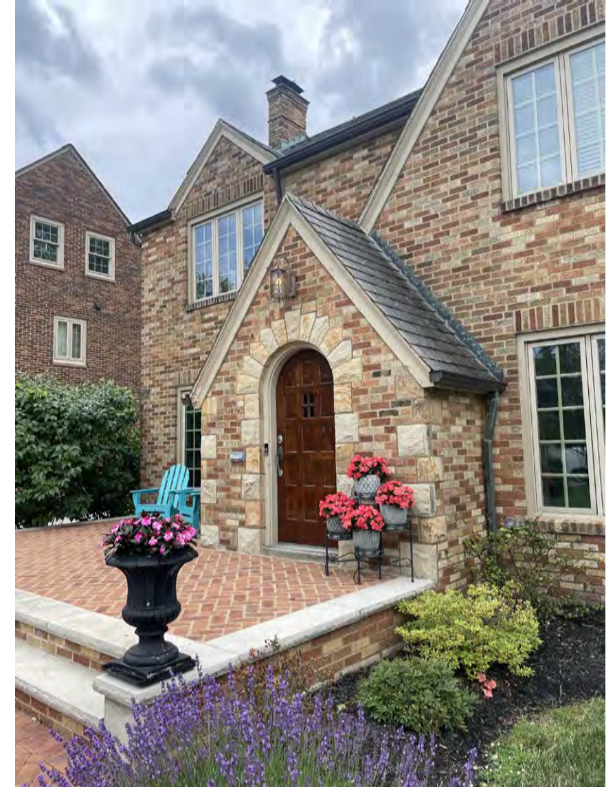
Existing Patio - From West
