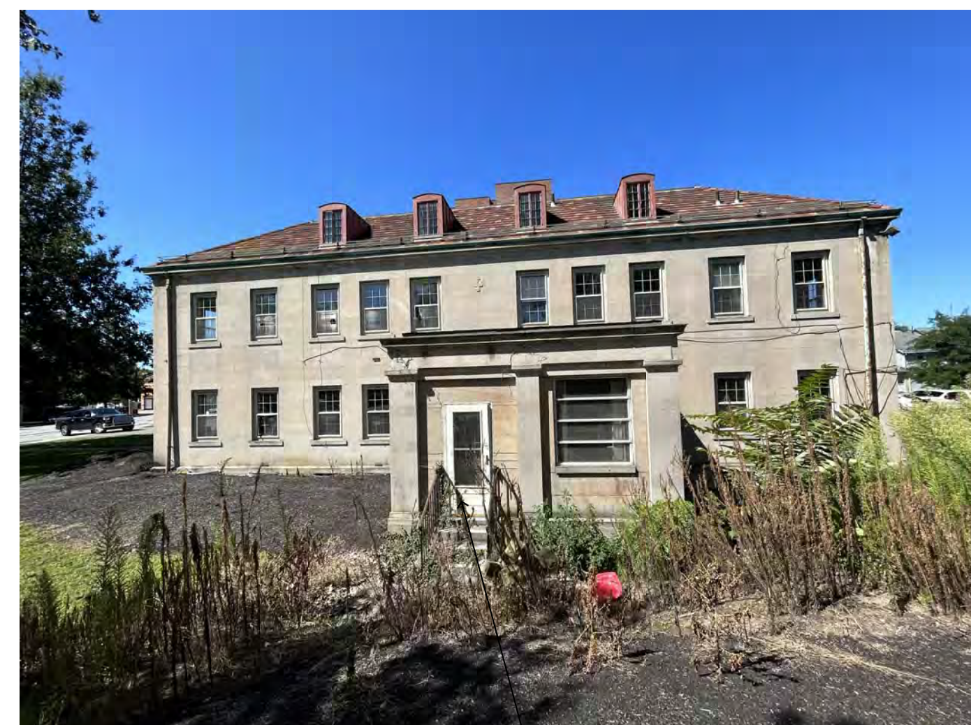
EAST ELEVATION AREA OF DOOR REMOVAL AND INFILL
