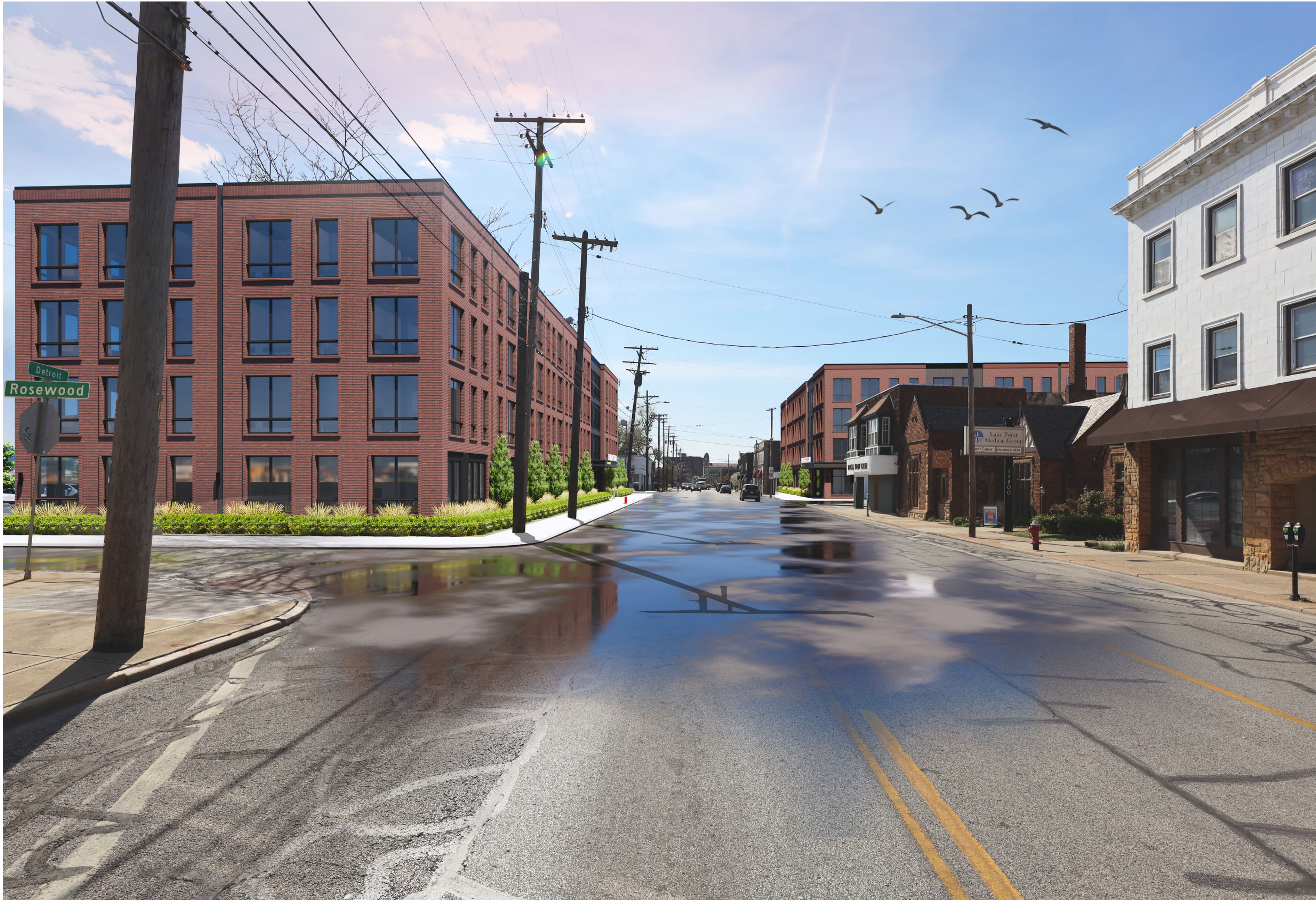
5. BUILDING NORTH & SOUTH - INTERSECTION OF ROSEWOOD AVENUE & DETROIT AVENUE
