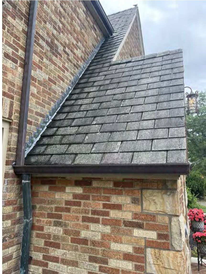
Existing Brick & Roofing
