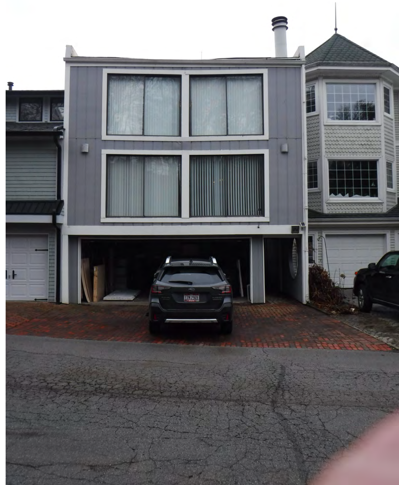
EXISTING CONDITIONS PHOTO VIEWING WEST N.T.S.
