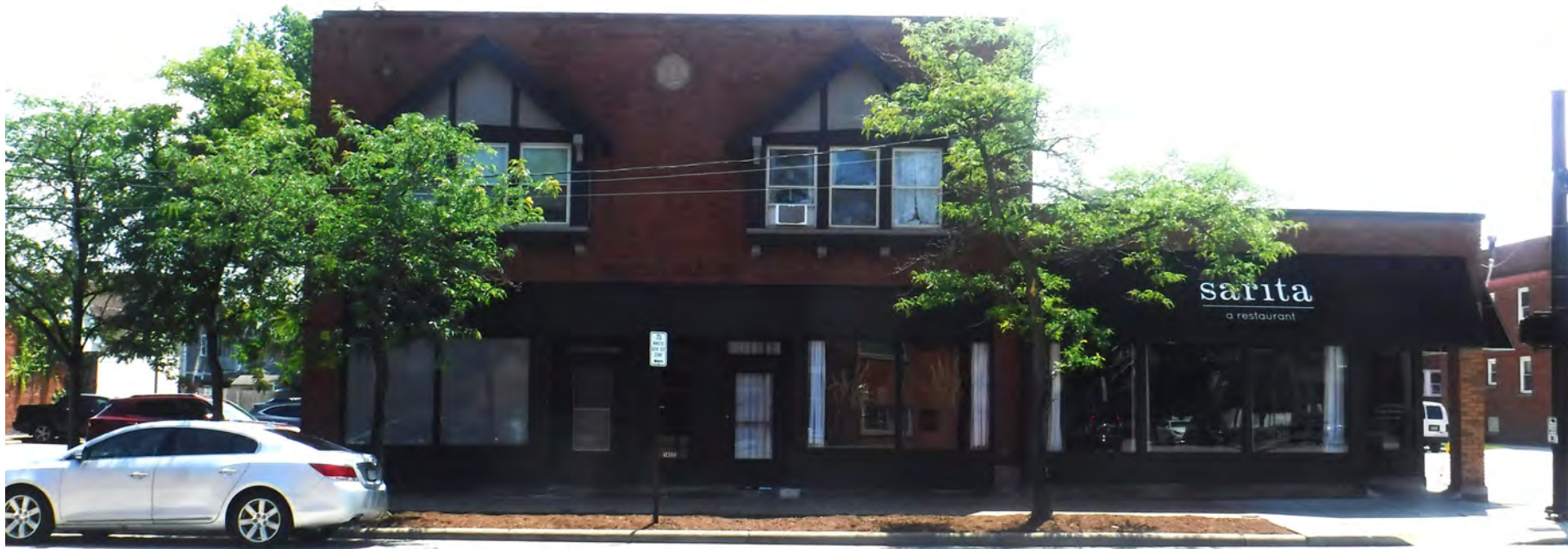
EXISTING CONDITIONS PHOTO VIEWING SOUTH N.T.S.
