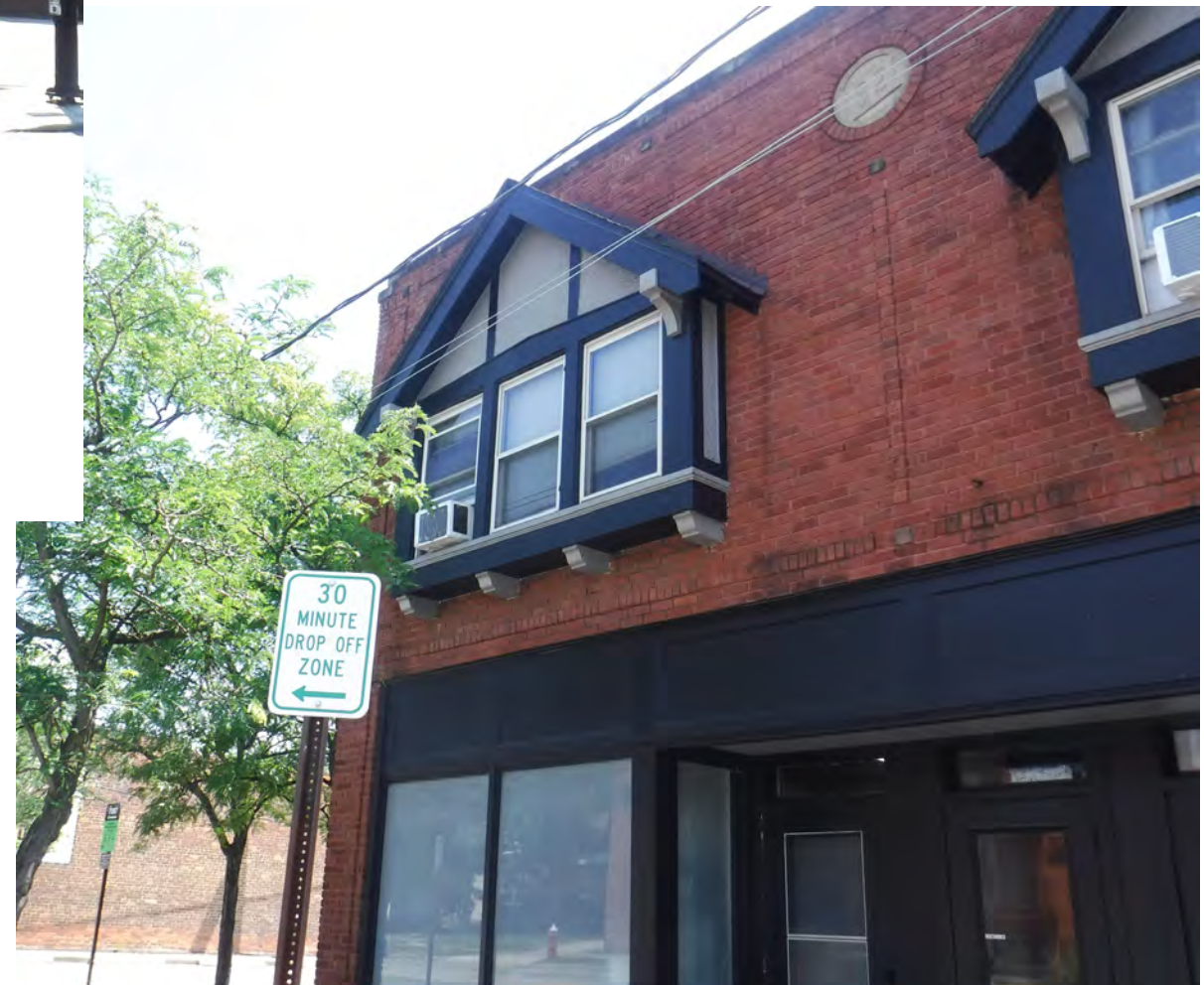
EXISTING CONDITIONS PHOTO VIEWING SOUTHEAST N.T.S.
