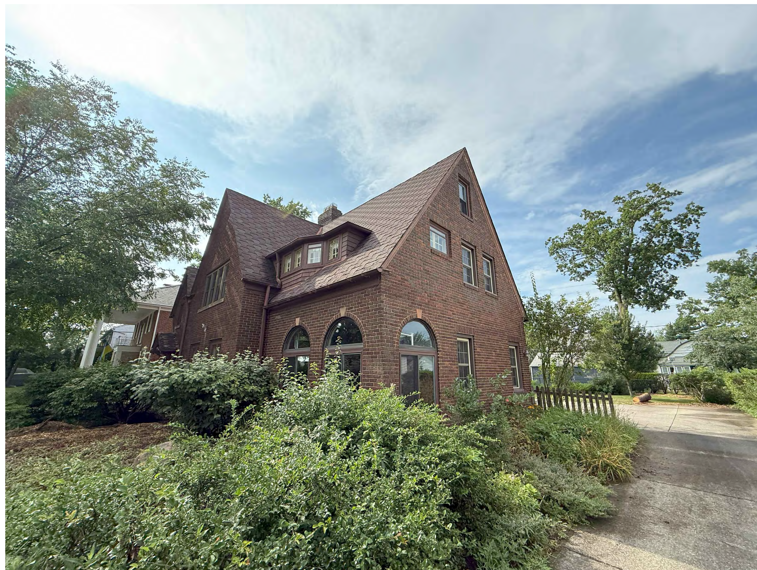
EXISTING HOUSE DORMER
