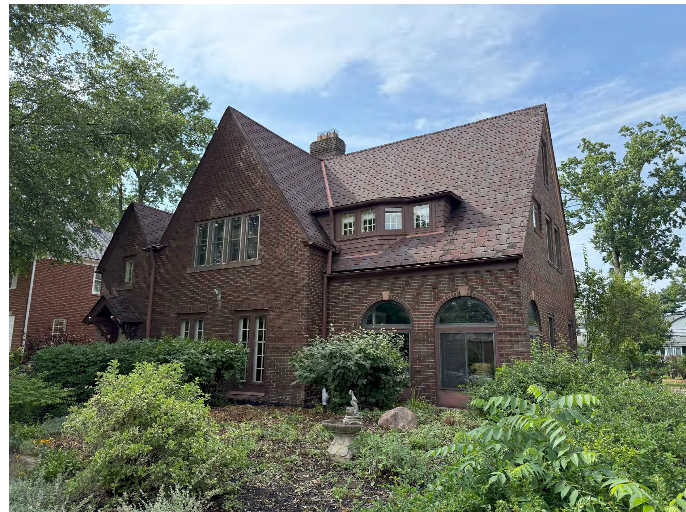
SOUTH FACE OF EXISTING HOUSE
