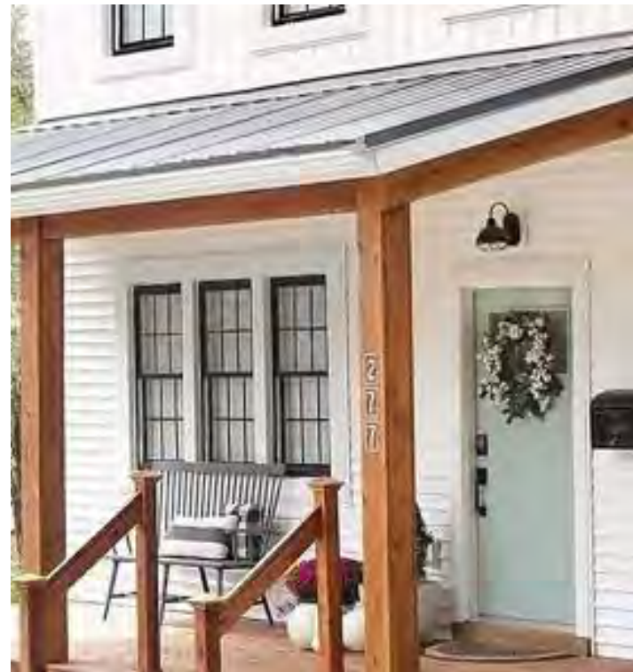
Wood Post and Metal Roof
