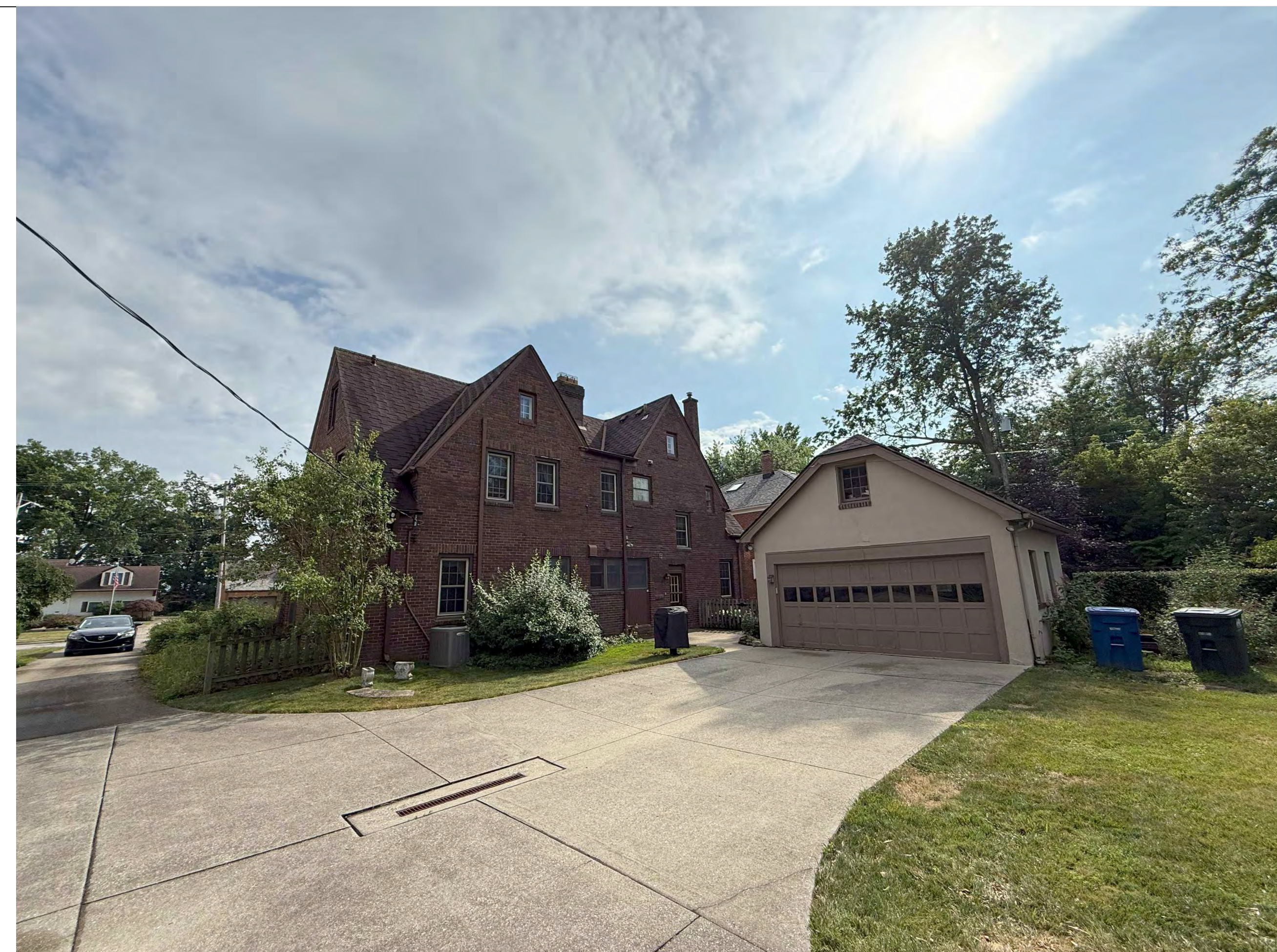
NORTH FACE OF EXISTING HOUSE
