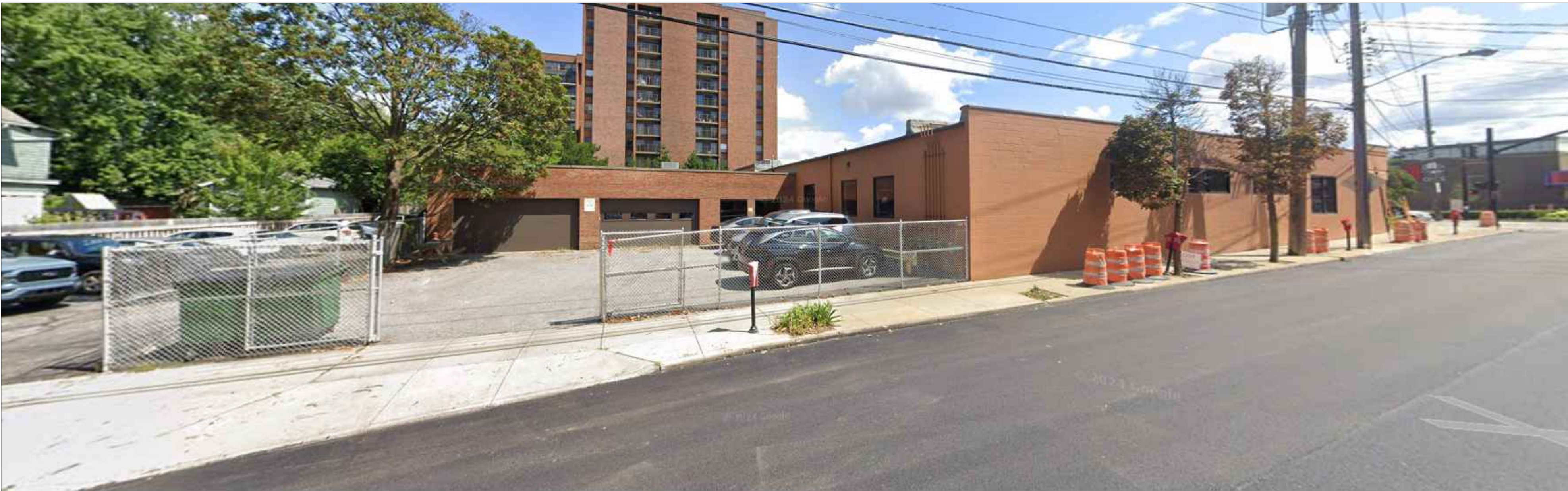
PHOTO OF EXISTING WEST ELEVATION
