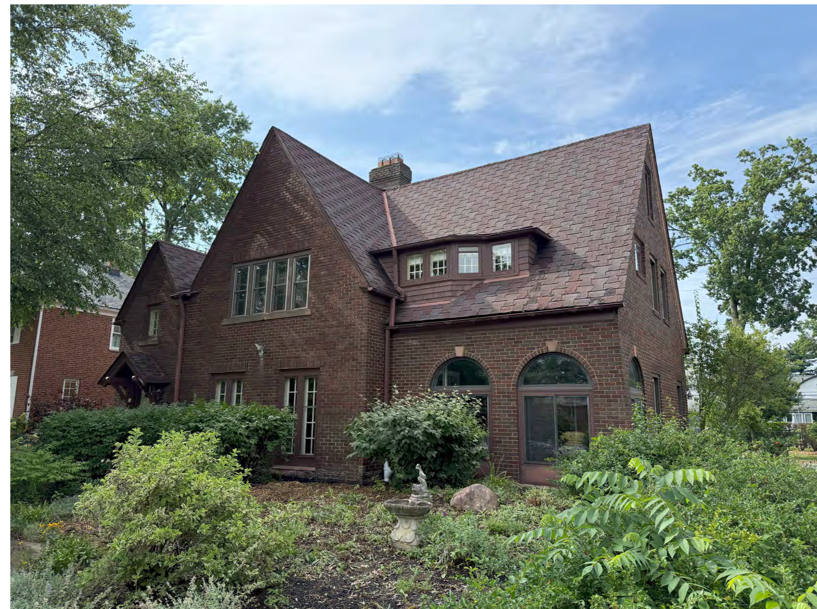
SOUTH FACE OF EXISTING HOUSE
