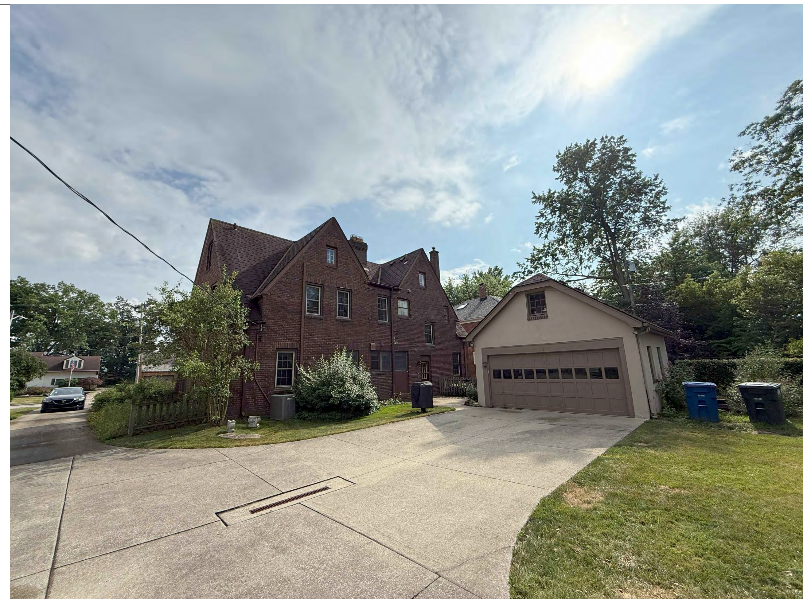
NORTH FACE OF EXISTING HOUSE
