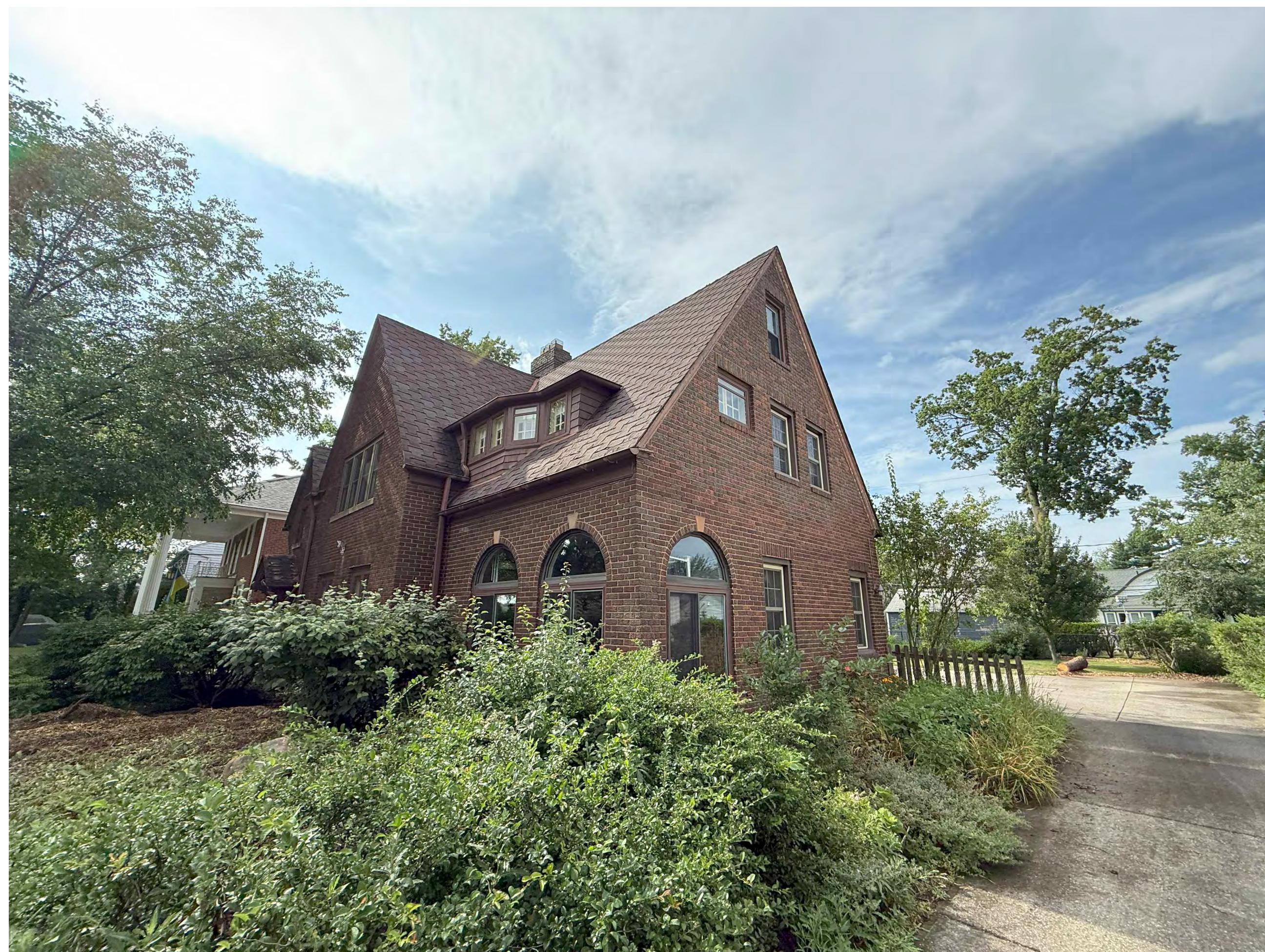
EXISTING HOUSE DORMER
