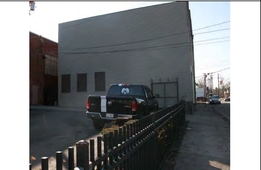
Photograph 4 – View of rear of property, looking south.
